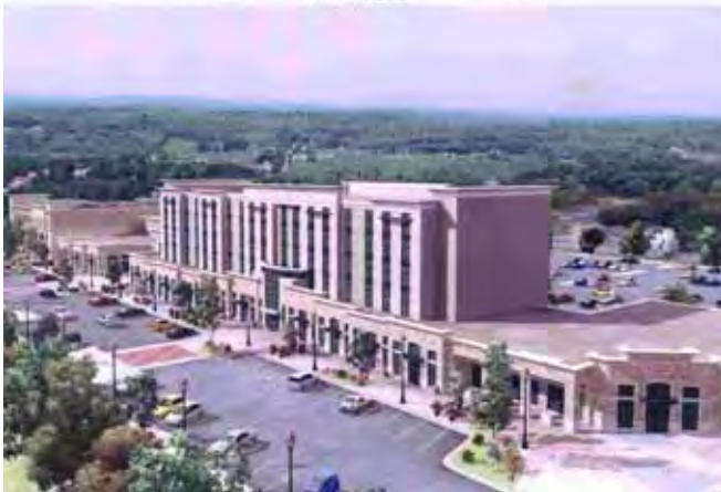
Colorado Street & 3rd Street - Looking SW
